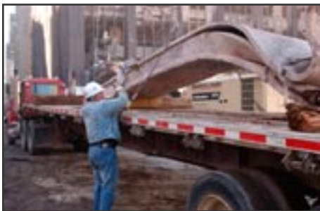
400 truck loads of steel per day were removed.
